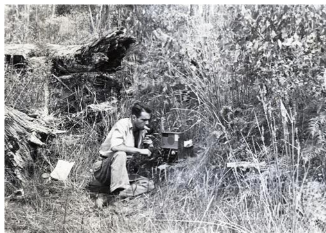
Portable RC-16B radios required a long wire strung up between the trees as an antenna. Source: FCRPA collection.
