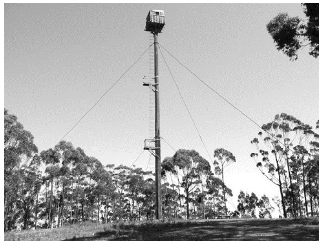
Stringer's knob tower near Orbost was built in 1941 at the suggestion of Herbert Duncan Galbraith, who was the Inspector of Forests in East Gippsland. The tower poles were 110ft long (100ft above the ground and 10ft below), with two trees - a yellow stringybark and a red ironbark bolted together. It had been listed on the Victorian Heritage Register but was sadly destroyed in the 2020 bushfires. Source: VHD
