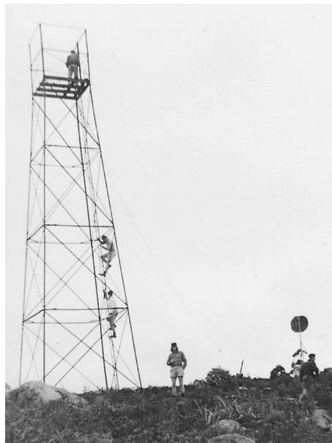
This rather flimsy looking structure is at Mt Disappointment. There are several references in FCV annual reports about using temporary scaffolding to test the suitability of sites before committing funds to major tower construction. This may be an example. Photo: Circa 1947 supplied by the Melbourne Walking Club. Source: Fire Lookouts Down Under.
