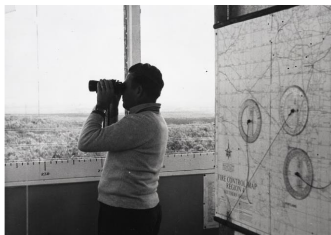
Frank Angilino, in the old fire tower at Sheoak Rise, north of Heywood, before it was moved by the FCV to a new site at Mt Annya in 1976. Note the map board with compass centres to triangulate and pinpoint the location of new fires. Source: FCRPA collection.
